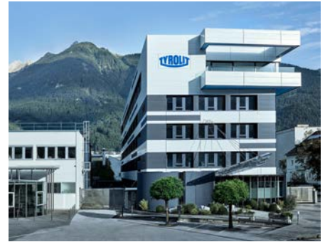
TYROLIT headquarters in Schwaz (Austria)
